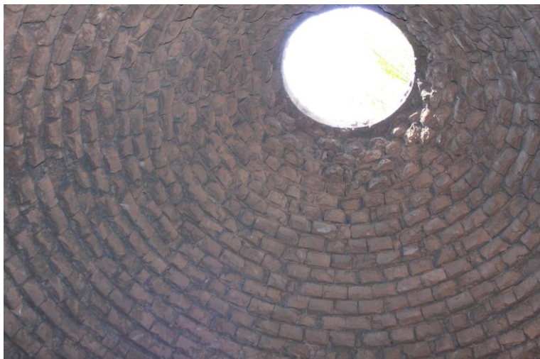
Figure 31. The interior of a coal-coal storehouse, Hadrovice village near Kacuni Source: Photos: Prof. Dr. Faruk Mekic (August 21, 2010)
