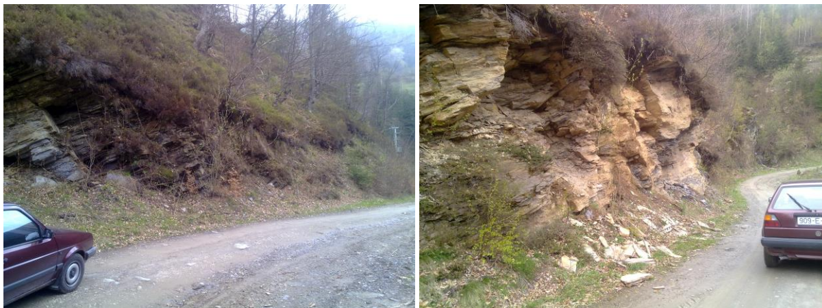
Figure 18. Natural stone (one of the basic building materials) Source: Author (April 17, 2011)
